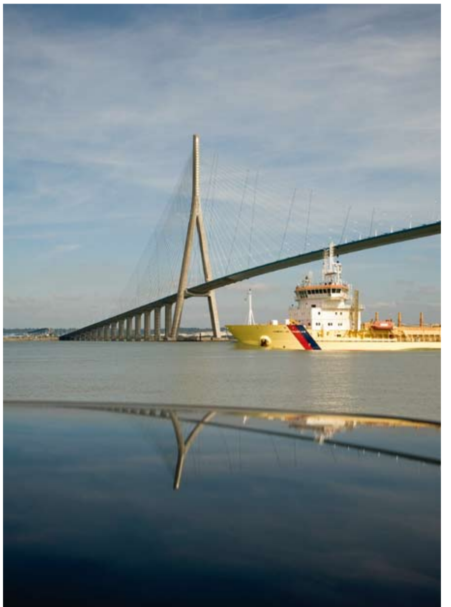
PONT DE NORMANDIE. When it opened in 1995, the Pont de Normandie was the world's longest cable-stayed bridge. The challenge was to span the mouth of the Seine River in one go, 50 meters above sea level, allowing the traffic below to move by unhindered.
